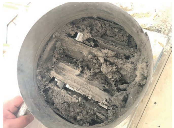
Figure 4: A heavily loaded duct.
