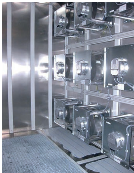
Figure 3: A fan wall in situ .
