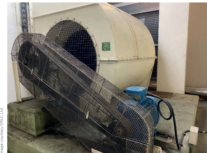
Figure 2: A large legacy belt-driven fan that could be replaced by a fan wall.
