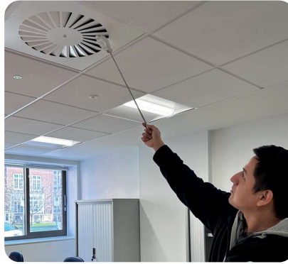
DRLC staff member Christian testing air flows for compliance.
